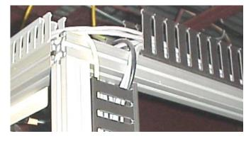
Figure 22: Wiring Channels
